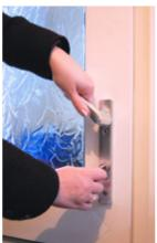
ALWAYS double-lock any UPVC doors by lifting the handle and locking it with the key to fully engage the security devices.
